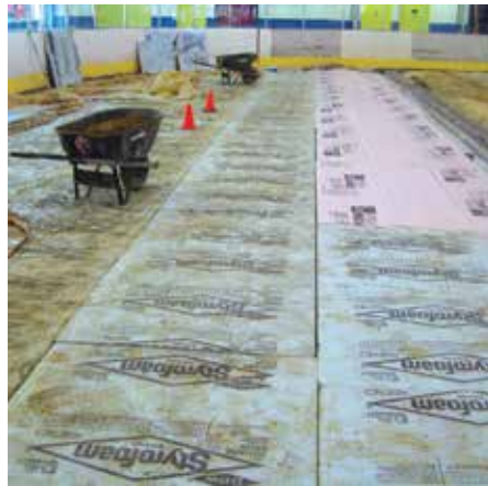
Rigid styrofoam insulation is installed below the secondary cooling piping.
